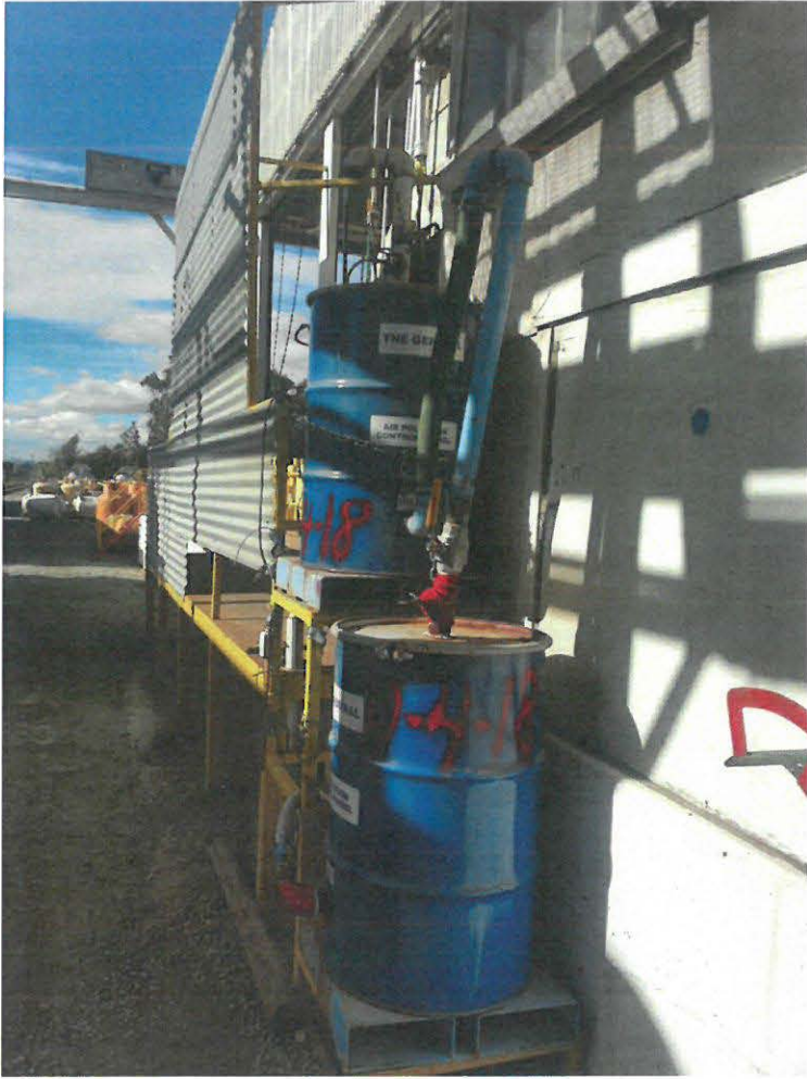
Figure 2. Carbon Drum Scrubber.
